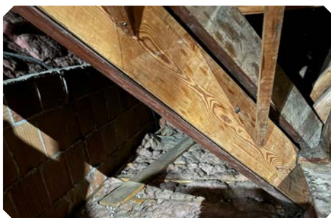
Top: attic dome. Bottom: gable.
